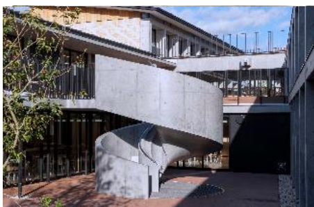
Air intake under spiral staircase
